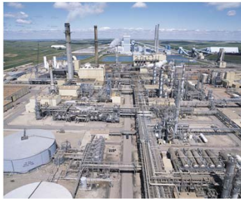
Dakota Gasification (Substitute natural gas plant in North Dakota) 达科他气化厂（北达科他州的替代天然气厂）
